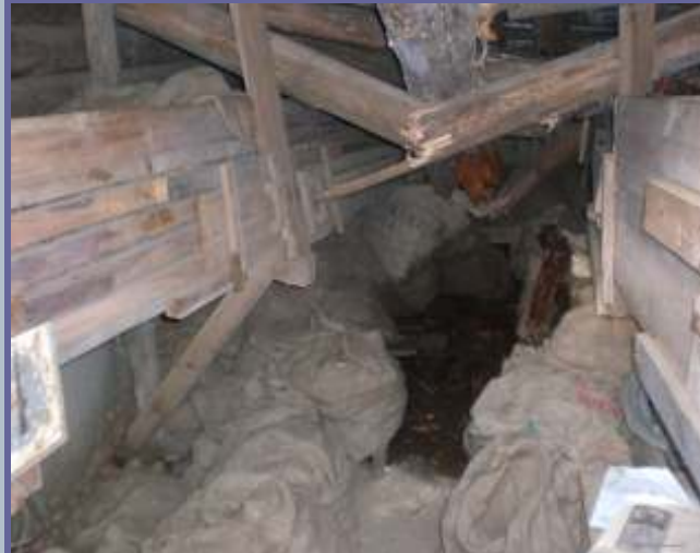
the disaster area of the former rootcellar
