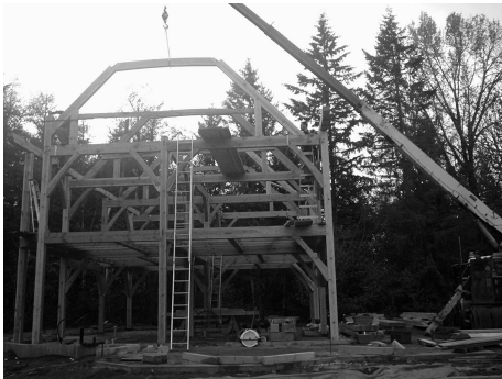
the raising of the frame
