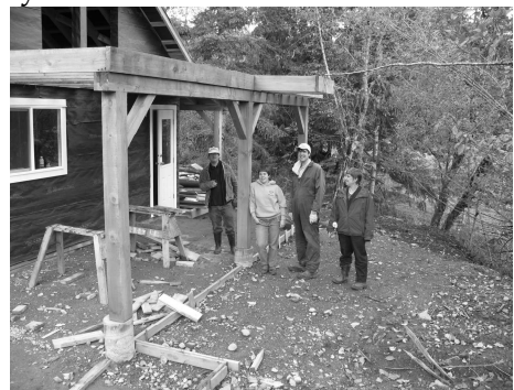
the utility building
